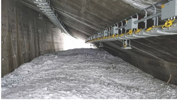
Figure 10. View inside U.S. Highway 550 snowshed filled with snow carried in from an avalanche on opposite side of the valley that pushed up onto the other side (highway side) of the valley. Snowshed is 18 km (11 mi) north of Silverton (Figure 7) (AIC/CDOT).
